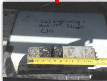
EAST 14TH STREET - CORE #10 HMA Layer 6" AB Layer 7" PCC Layer 5.5"
