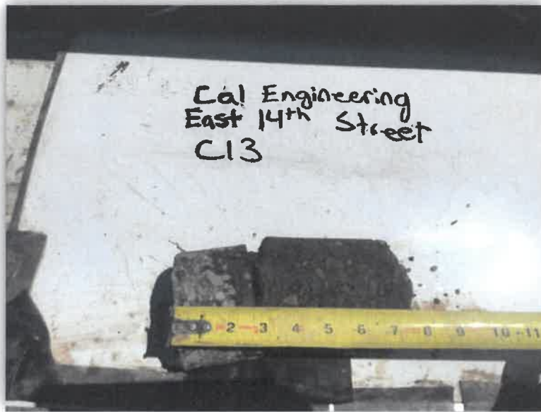
EAST 14TH STREET - CORE #13 HMA Layer 8" AB Layer 0" PCC Layer 0"
