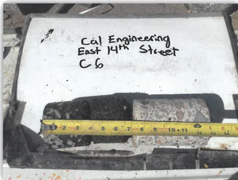
EAST 14TH STREET - CORE #6 HMA Layer 7" AB Layer 0" PCC Layer 6"
