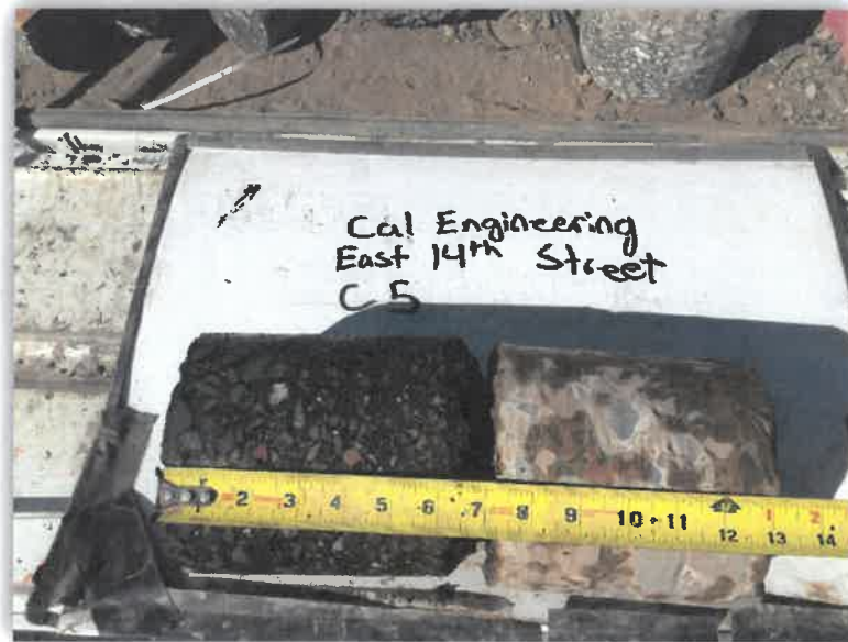
EAST 14TH STREET - CORE #5 HMA Layer 7.5" AB Layer 0" PCC Layer 6"
