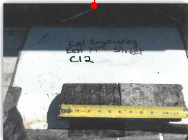
EAST 14TH STREET - CORE #12 HMA Layer 6" AB Layer 2.5" PCC Layer 6"
