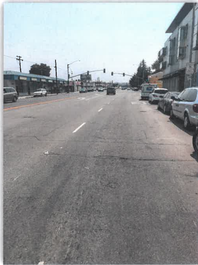
EAST 14 TH STREET – LOCATION #2 Near Kent Street SB
