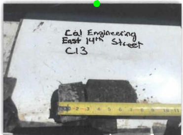
EAST 14TH STREET - CORE #13 HMA Layer 8" AB Layer 0" PCC Layer 0"
