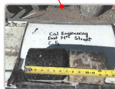
EAST 14TH STREET - CORE #5 HMA Layer 7.5" AB Layer 0" PCC Layer 6"
