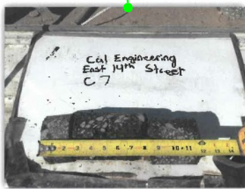
EAST 14TH STREET - CORE #7 HMA Layer 12" AB Layer 0" PCC Layer 0"
