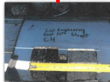
EAST 14TH STREET - CORE #4 HMA Layer 6" AB Layer 8" PCC Layer 4.5"
