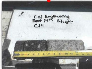
EAST 14TH STREET - CORE #14 HMA Layer 6.5" AB Layer 3" PCC Layer 7"
