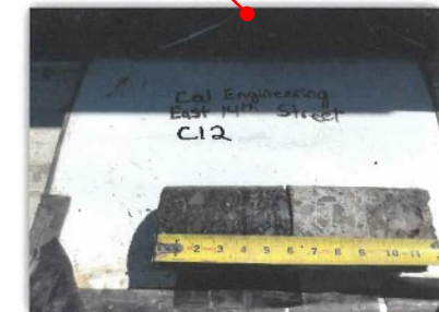
EAST 14TH STREET - CORE #12 HMA Layer 6" AB Layer 2.5" PCC Layer 6"
