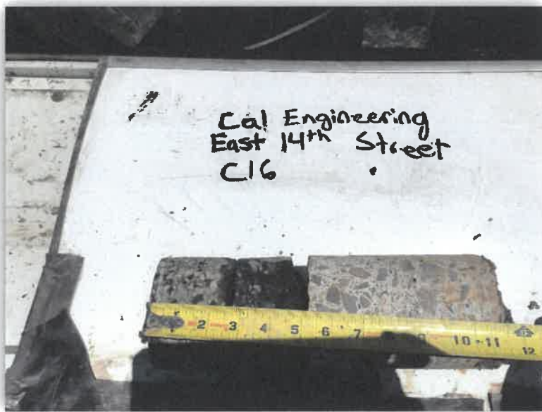
EAST 14TH STREET - CORE #16 HMA Layer 5.5" AB Layer 3" PCC Layer 6.25"
