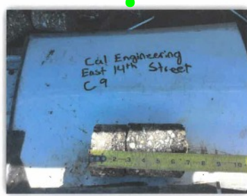
EAST 14TH STREET - CORE #9 HMA Layer 6.75" AB Layer 7" PCC Layer 0"
