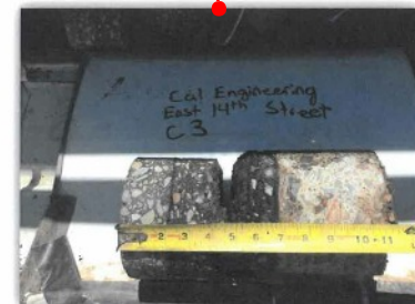
EAST 14TH STREET - CORE #3 HMA Layer 6.5" AB Layer 0" PCC Layer 5"
