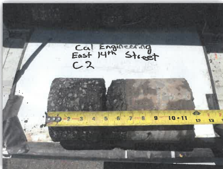
EAST 14TH STREET - CORE #2 HMA Layer 6.5" AB Layer 0" PCC Layer 5.5"
