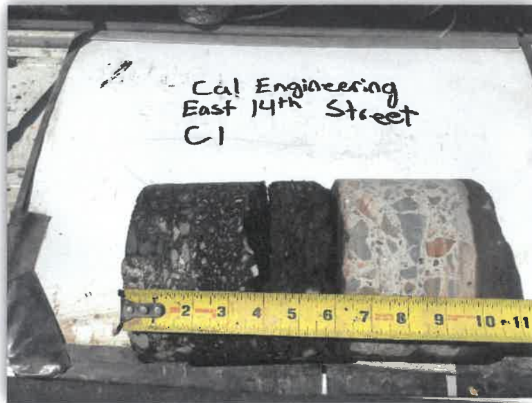
EAST 14TH STREET - CORE #1 HMA Layer 6" AB Layer 0" PCC Layer 4.5"
