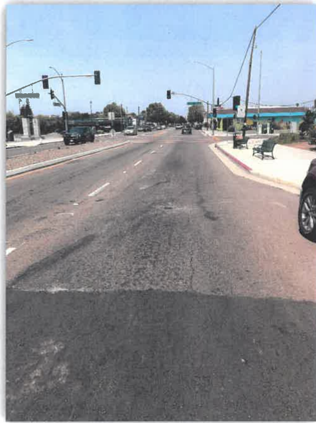
EAST 14 TH STREET – LOCATION #8 Near 163 rd NB
