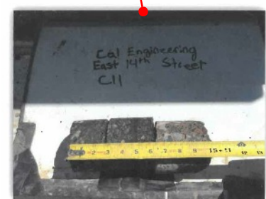
EAST 14TH STREET - CORE #11 HMA Layer 6" AB Layer 5" PCC Layer 4"
