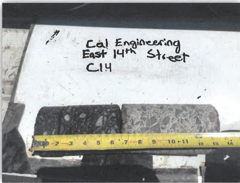
EAST 14TH STREET - CORE #14 HMA Layer 6.5" AB Layer 3" PCC Layer 7"
