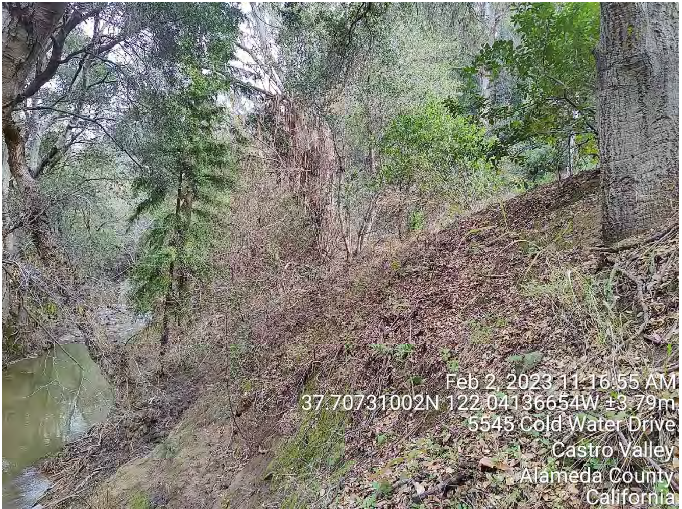
Photograph 2. Slope Below Boring A-23-001 Location
