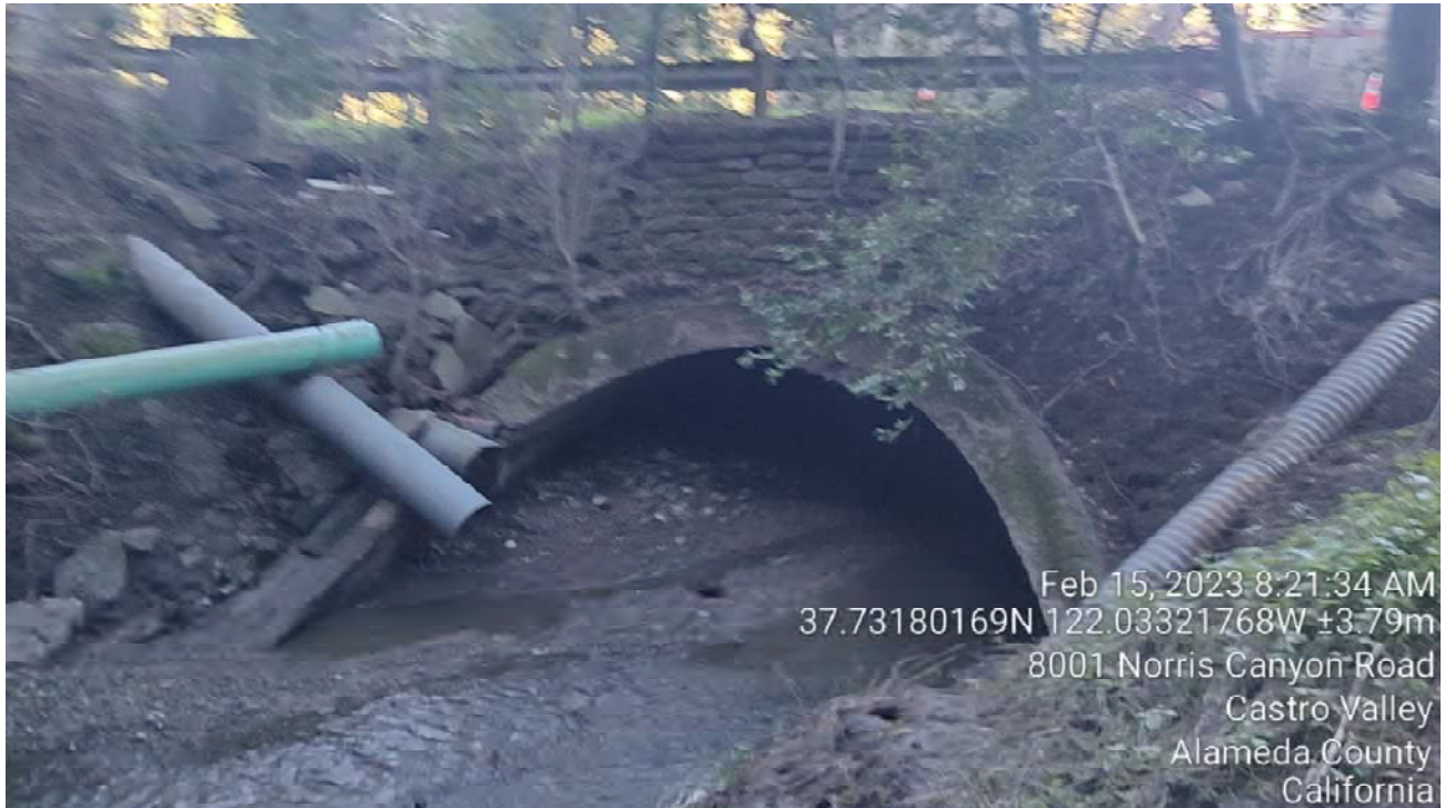
Photograph 16. Culvert Inlet South of Boring A-23-008 Location
