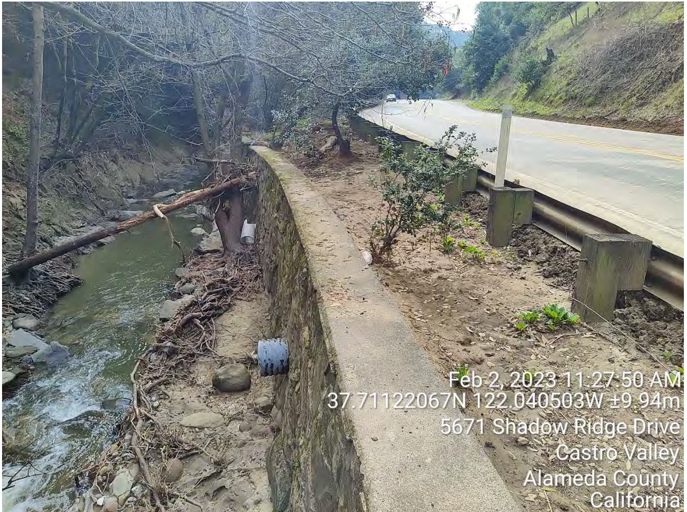
Photograph 5. Retaining Wall Adjacent to Northern End of South Guardrail, Looking South
