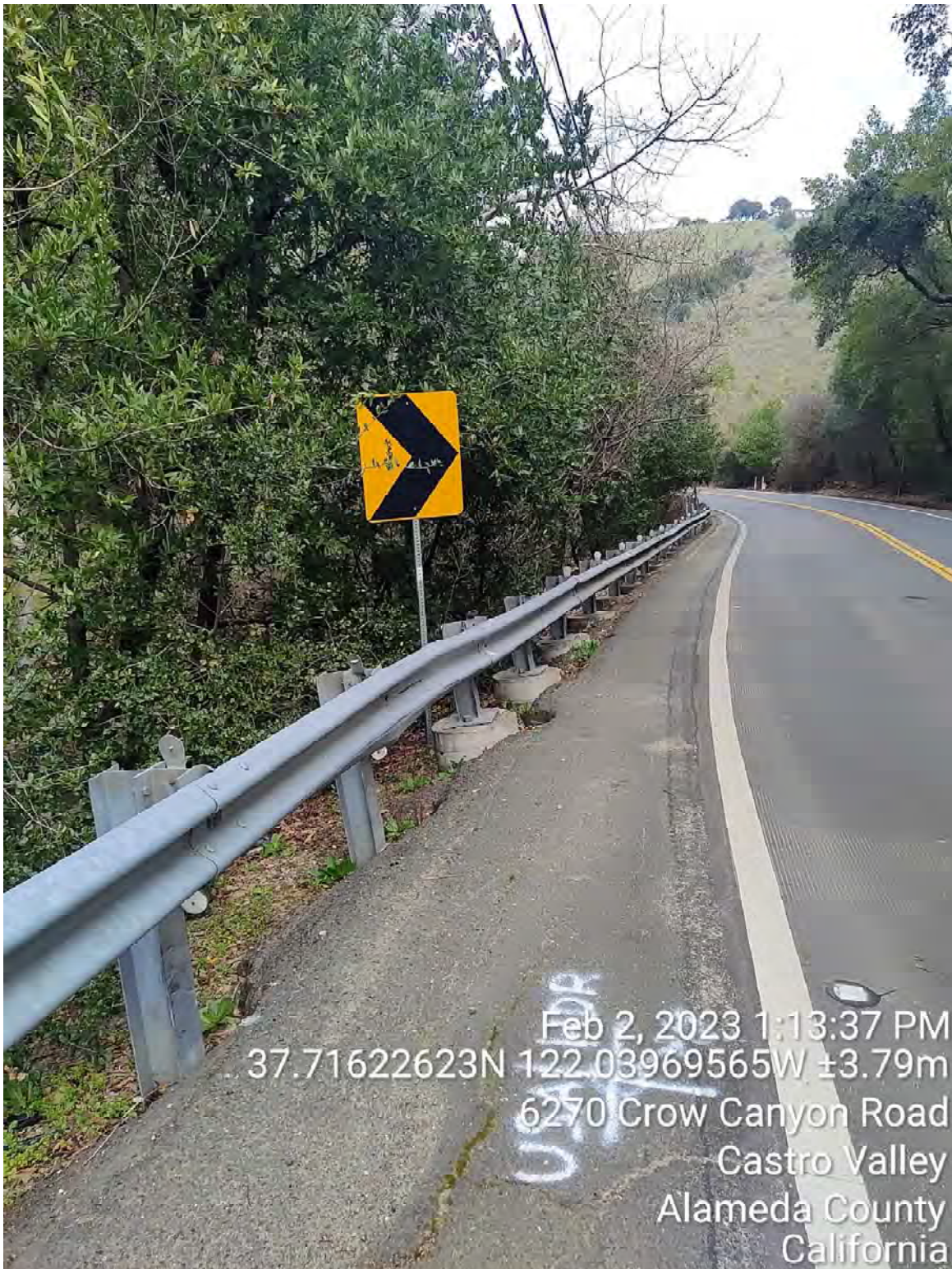
Photograph 8. Guardrail North of Boring A-23-004 Looking North-Northeast
