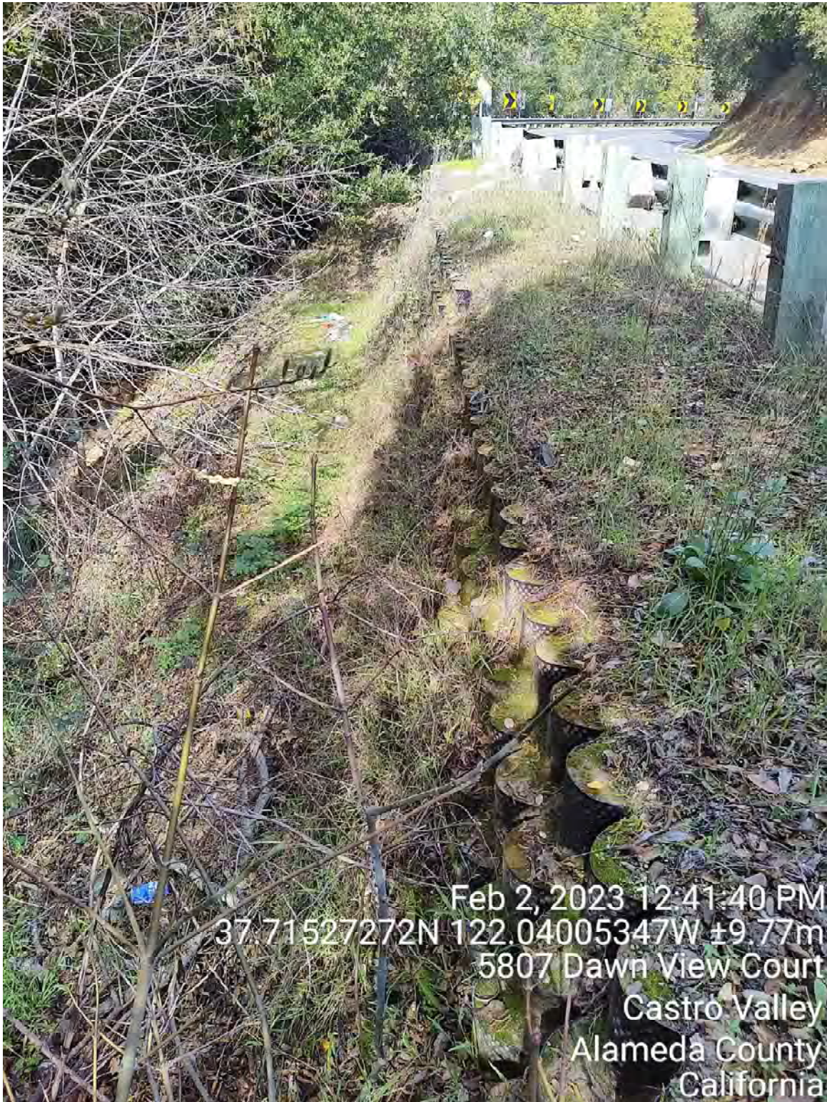
Photograph 6. Mechanical Stabilized Earthen Wall West of Existing Guardrail, Looking North
