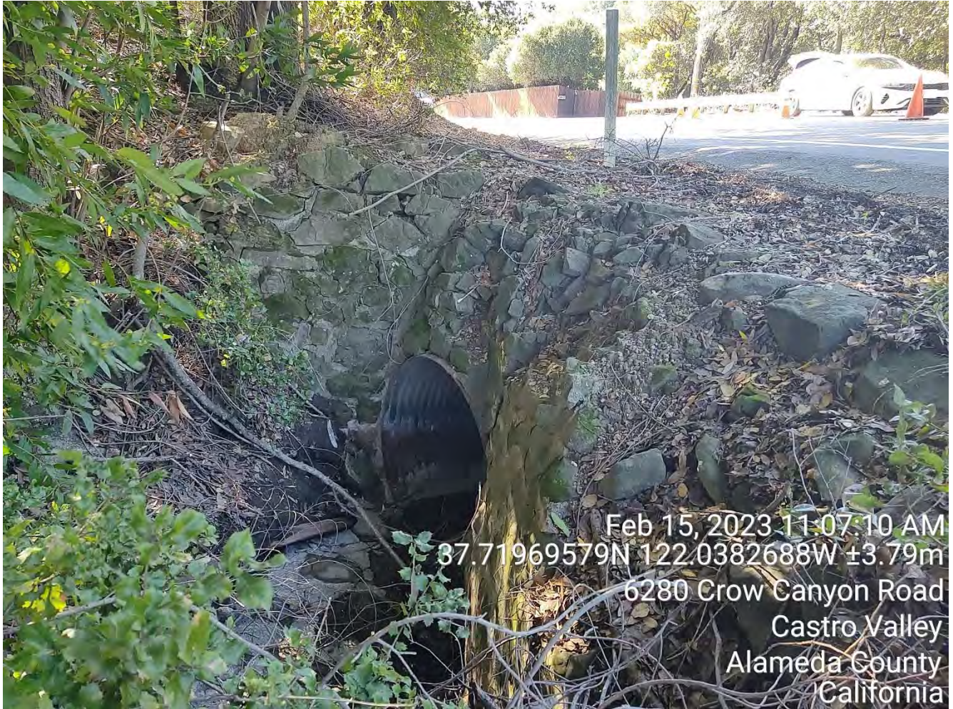
Photograph 15. Culvert Inlet Adjacent to Guardrail No. 6 Segment Looking Southwest
