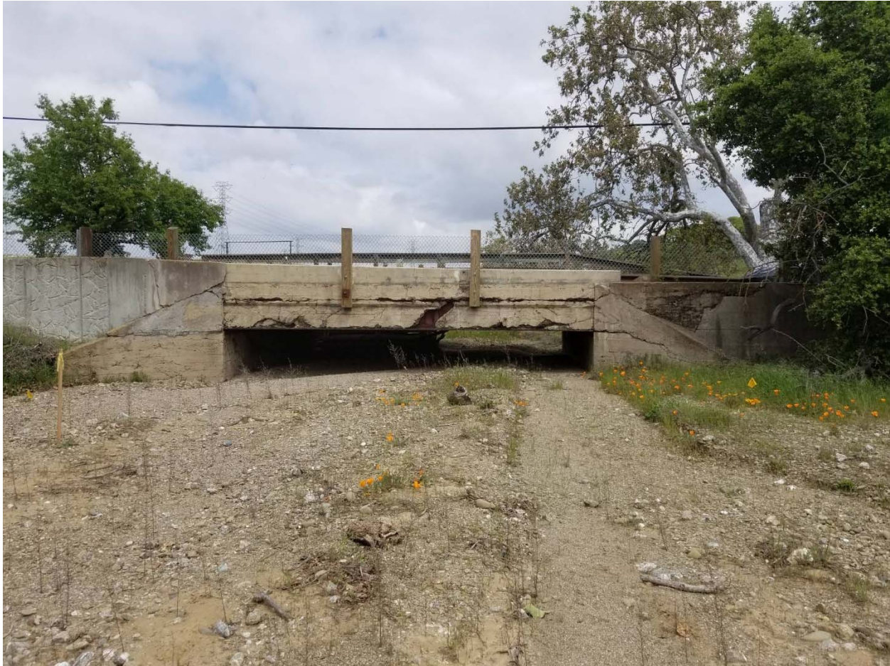
Photo 2. Downstream Face of Existing Bridge (April 10, 2020)
