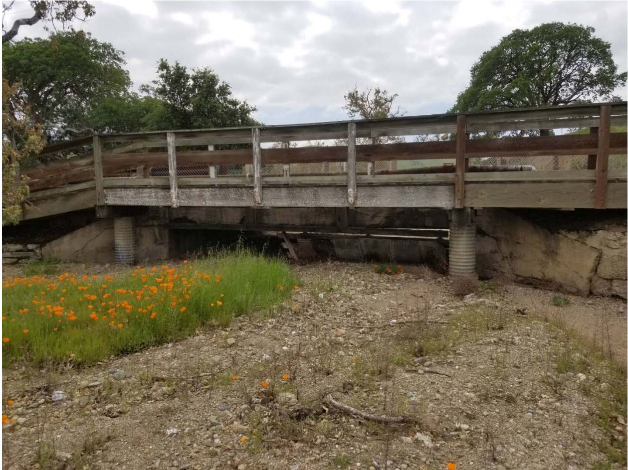
Photo 1. Upstream Face of Existing Bridge (April 10, 2020)
