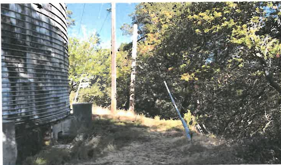
Figure 2b Surrounding Vegetation at the Castlewood Tank Replacement Site
