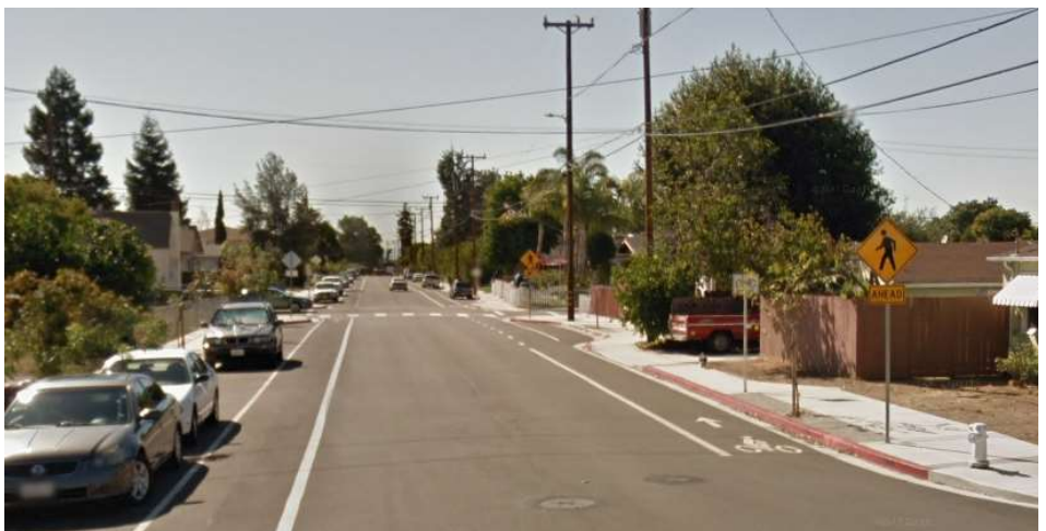
Figure D.2. A Class II bike lane along Grove Way Between Meekland Avenue and Western Boulevard in Cherryland
