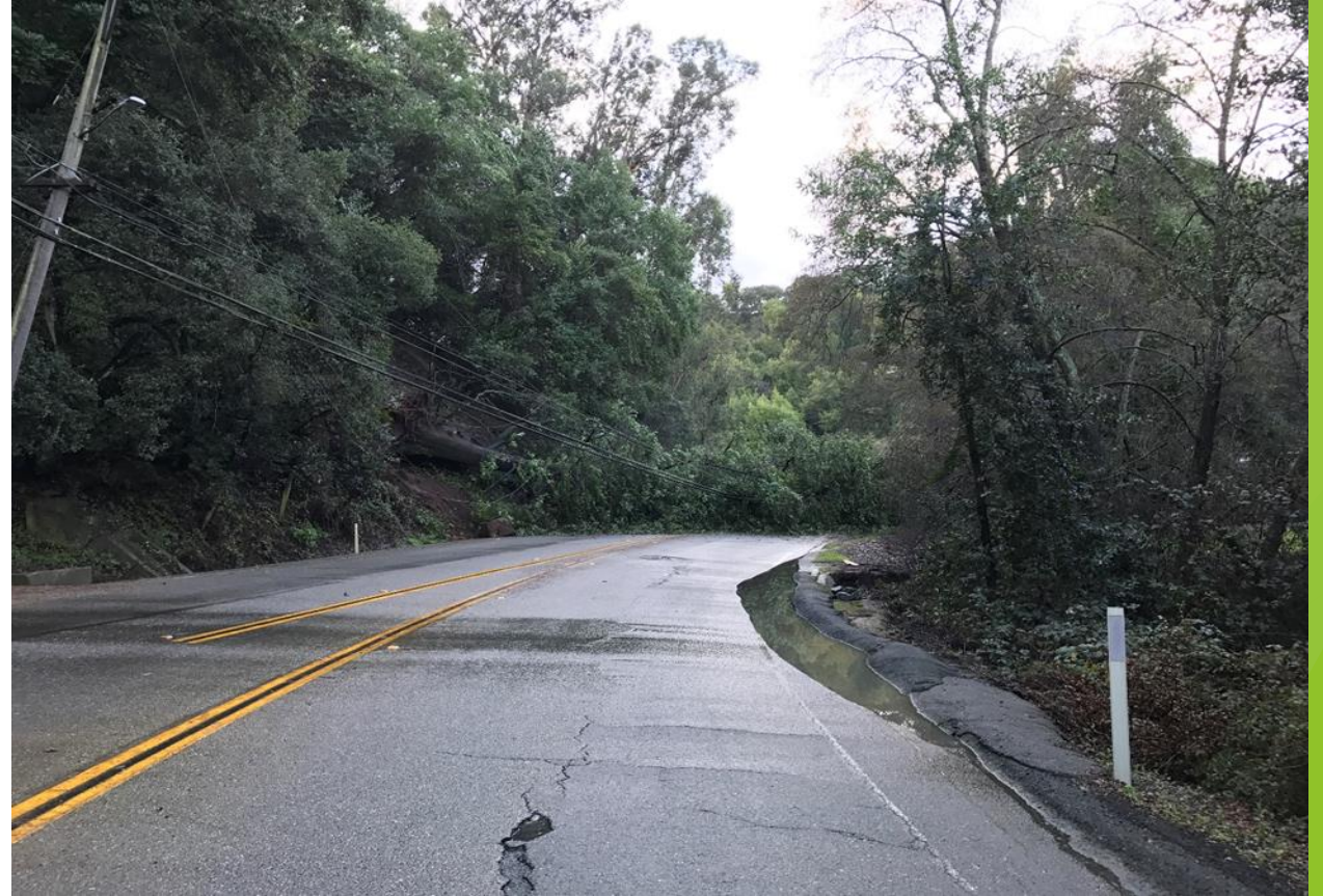
Crow Canyon Road, between Greenridge Road and Norris Canyon Road, Castro Valley. Large Bay tree fell, taking power lines with it.
