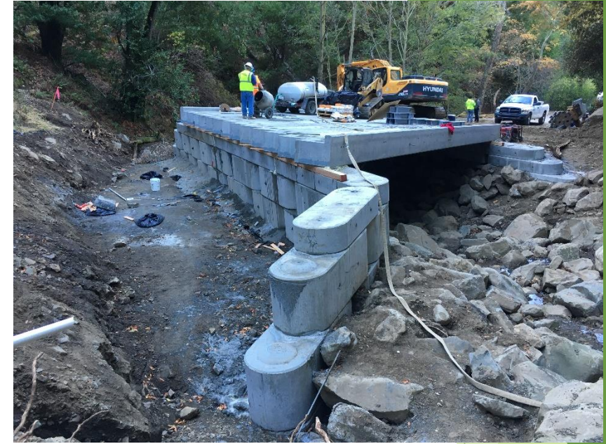
Stonybrook Creek Bridge Palomares Road
