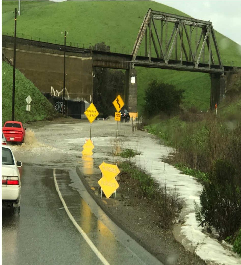
Altamont Pass Road Flooding
