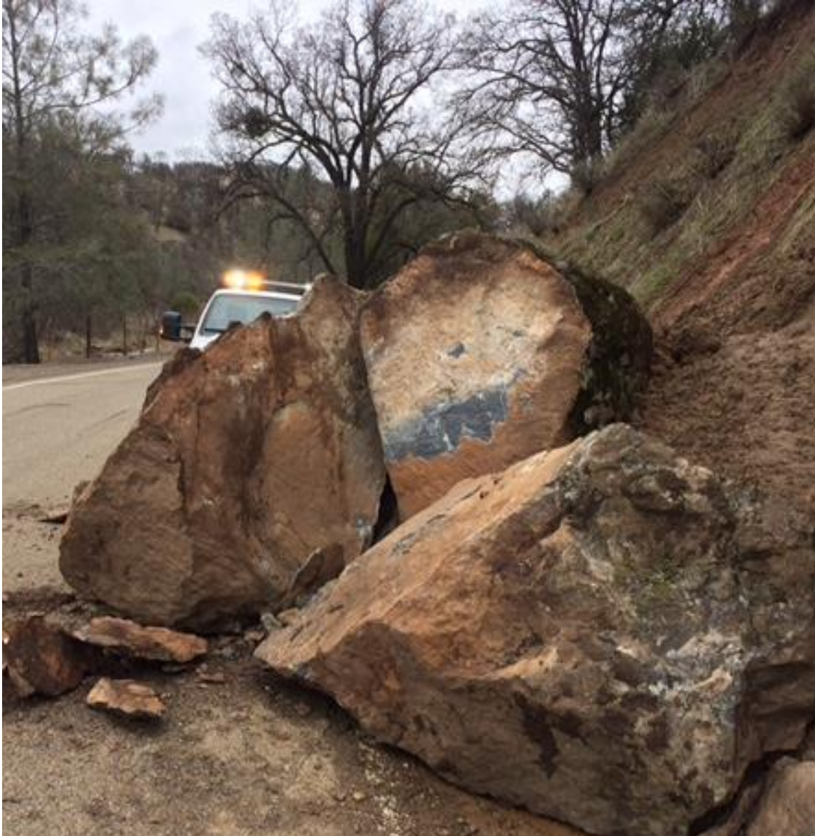
Mines Road Slip-Out
