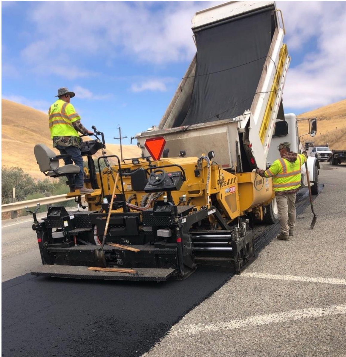
Altamont Pass Road Pavement Patching
