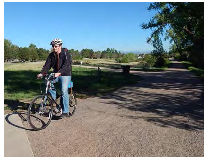
High Line Canal Trail - a crusher fines path free of ruts and weeds
