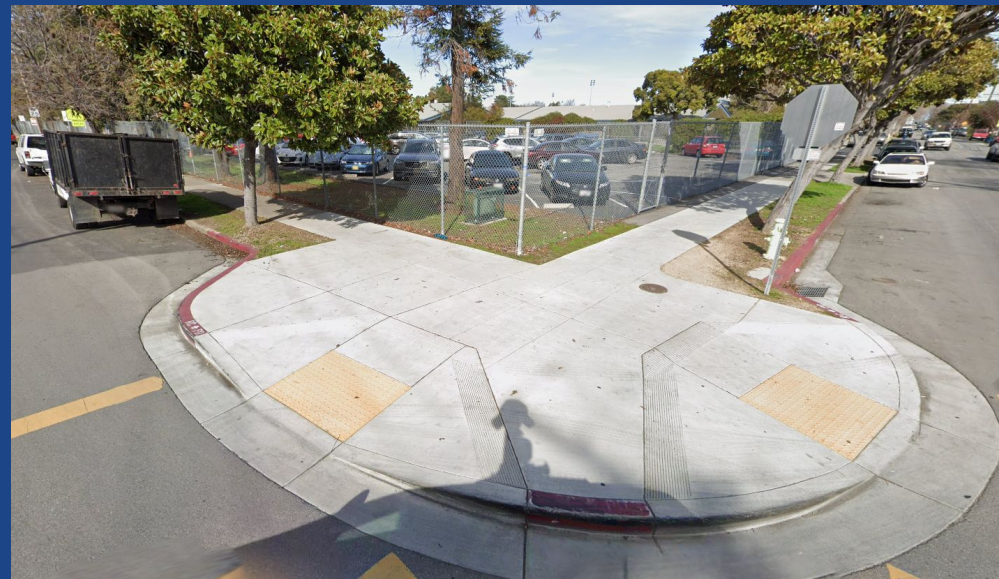
Two Curb Ramps at Each Corner
