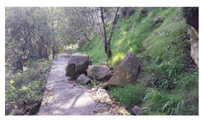
Localized rockslides are common within the steeper sections of the Canyon; here rocks fell atop the Sunol Aqueduct east of the Farwell Bridge
