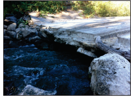
Figure 2-9 Weir Undermining
