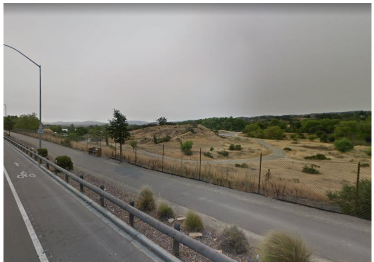
Figure 5.4. Example of shared use path adjacent to Stanley Boulevard in the Tri-Valley area
