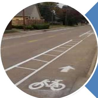
**Buffered Bicycle Lanes (Class II)** are implemented by painting or otherwise creating a flush buffer zone between a bicycle lane and the adjacent travel lane. While buffers are typically used between bicycle lanes and motor vehicle travel lanes, they may also be installed between bicycle lanes and parking lanes.
