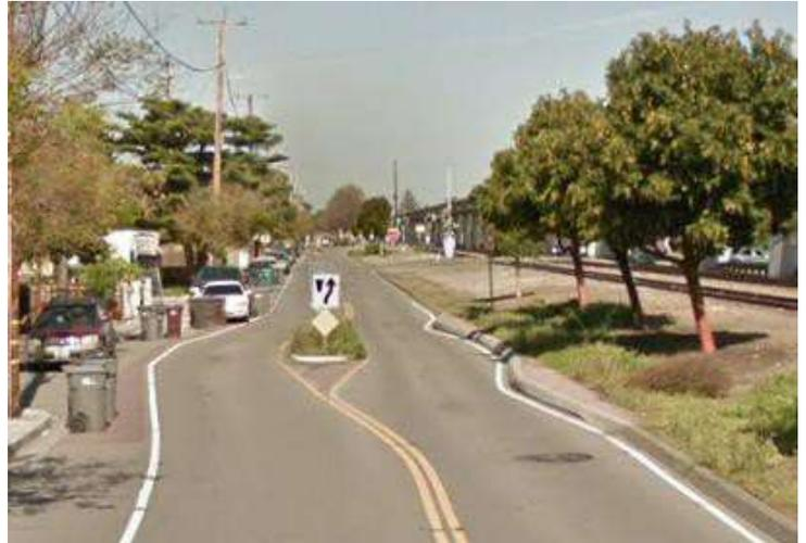
Figure 5.5. Example of center island treatment to horizontally deflect traffic and reduce speeds on Western Blvd in Cherryland
