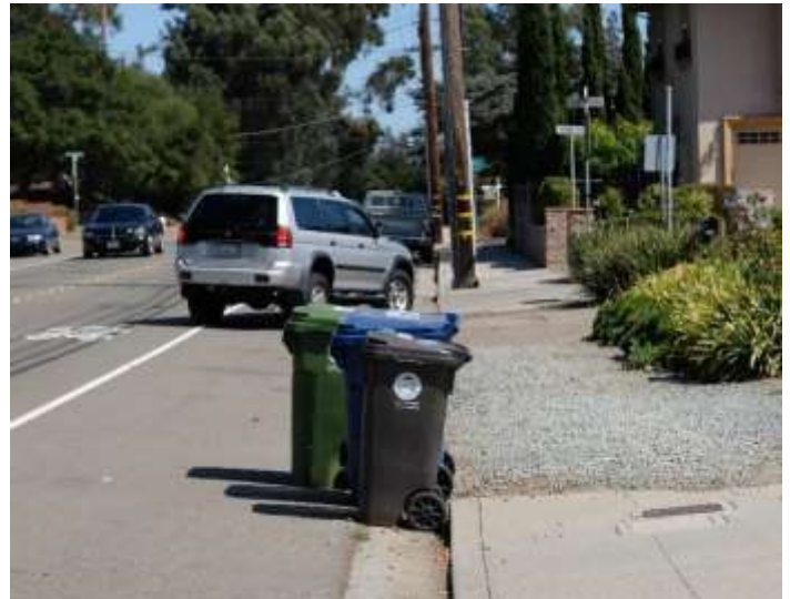
Figure 5.1. Opportunity to fill in sidewalk gap on Heyer Ave in Castro Valley
