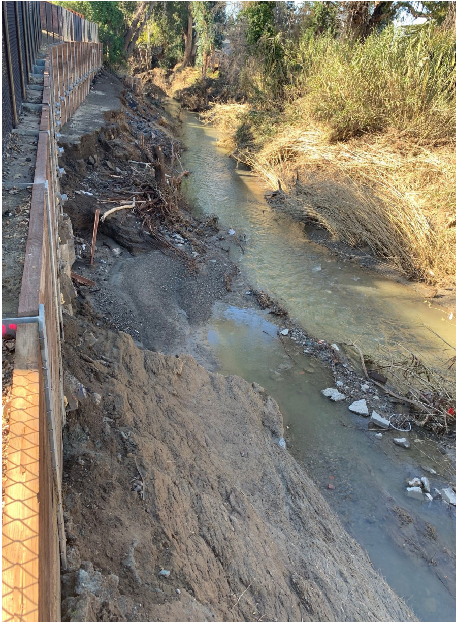
San Lorenzo Creek behind Wingate Way Creek bank washed out undermining retaining wall
