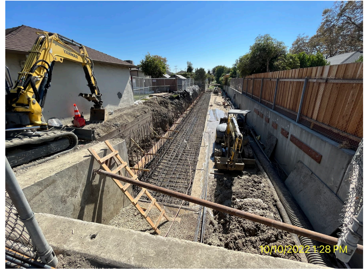
Estudillo Canal Channel Wall Reconstruction
