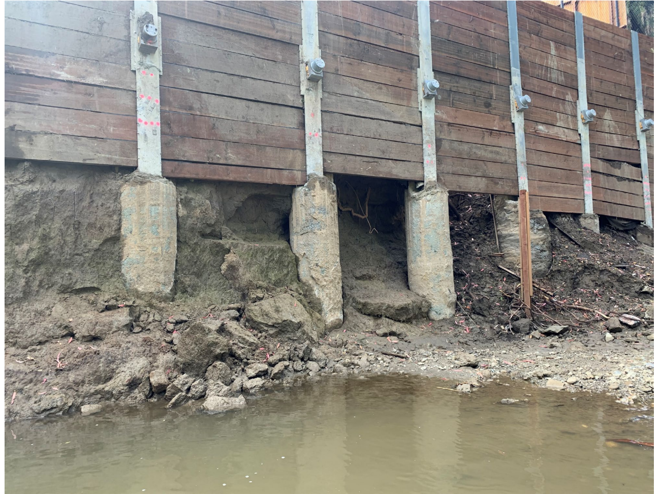
San Lorenzo Creek behind Wingate Way Creek bank washed out undermining retaining wall
