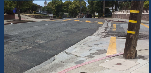
Faded crosswalks and striping
