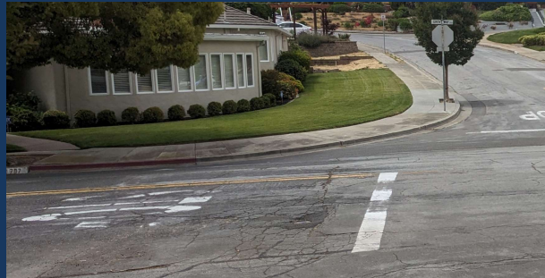
Missing curb ramps
