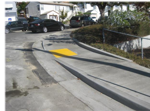
ADA compliant curb ramps
