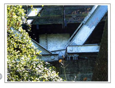
Figure 21: Farwell Bridge truss ends supported by 1896 additional pier. October, 2003.
