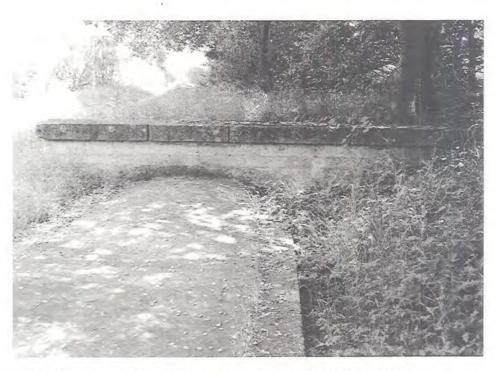
Above and below: Two views of box flume aqueduct connections to headwalls of aqueduct tunnels.
